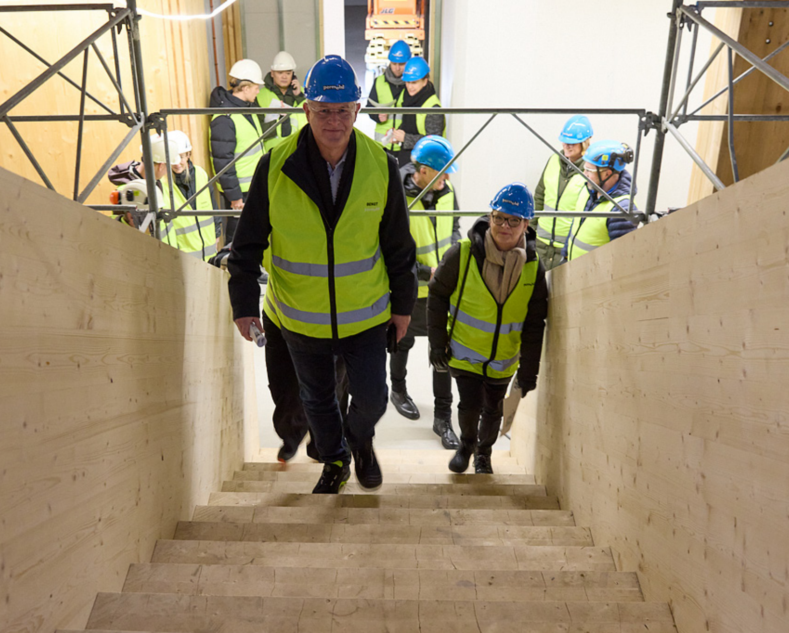
Building continues on our new facility in Västernorrland, Sweden.
